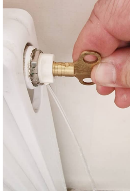
BLEEDING A RADIATOR
